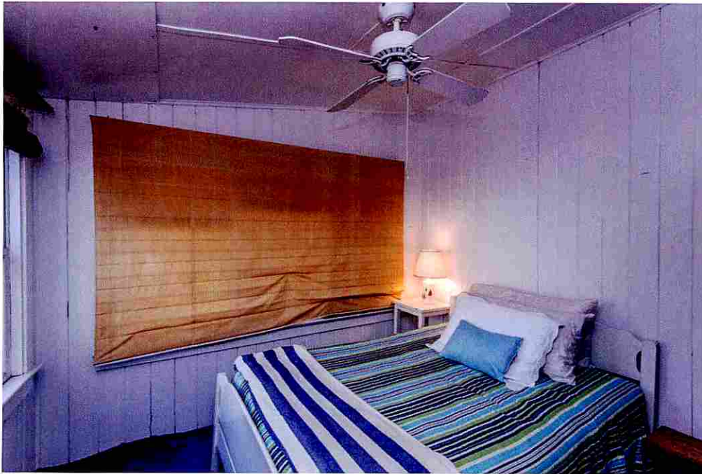
Figure 7. The above pictures shows the second floor fill south of the kitchen to create a second bedroom on the main level. No hardwoods are visible, paneling and windows do not match the existing original architectural fabric.
