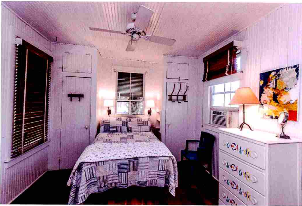
Figure 5. Original southern second floor bedroom with two closets shows the original simplistic wall and ceiling paneling and trim that still existing throughout the original structure along with the hard pine flooring, which no longer exists in the kitchen only.
